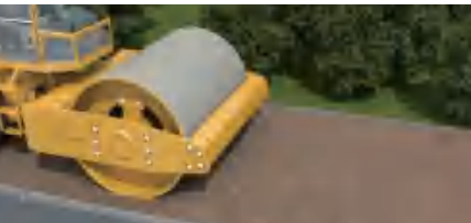
01 Ground base preparation
