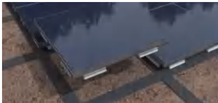
03 Install PV floor tiles
