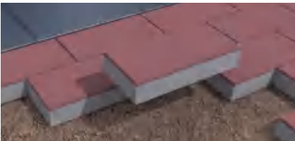
05 Laying surrounding materials
